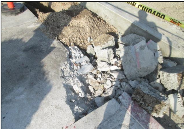
Broken Existing SW at Sta 70+29.13
