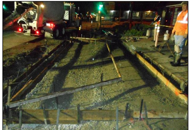
Forms Set at DW Sta. 65+72.61
