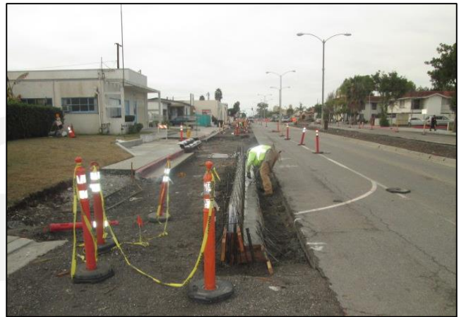
Finishing Curb and Gutter
