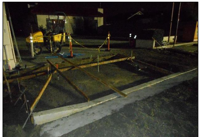
Forms Set and Ready for 5500 PSI PCC at Sta 70+29.13
