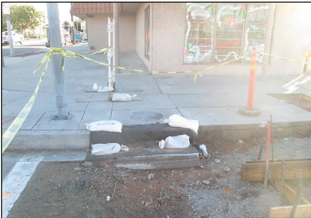
Closed Catch Basin BMP
