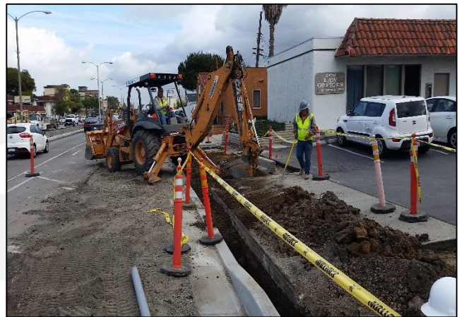
Demolition of Existing Driveway
