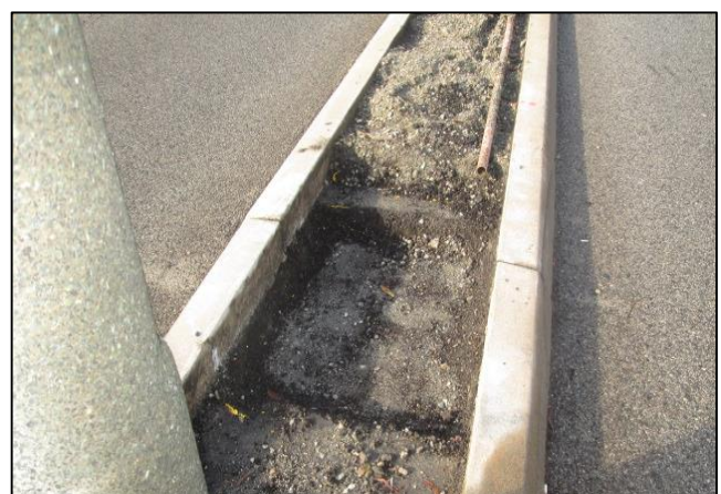
Pavement Removed for Street Light Base at Sta 57+09
