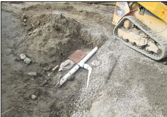
Y fitting Replaced per Bldg. Inspector
