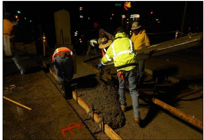
Placing 5500 PSI PCC at driveway 67+26.28
