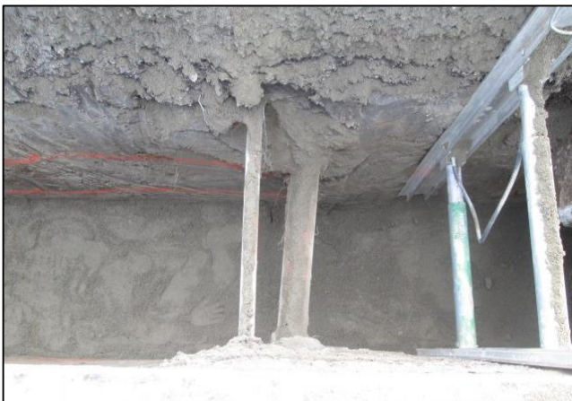
Two Unmarked Lines at Sta 73+50
