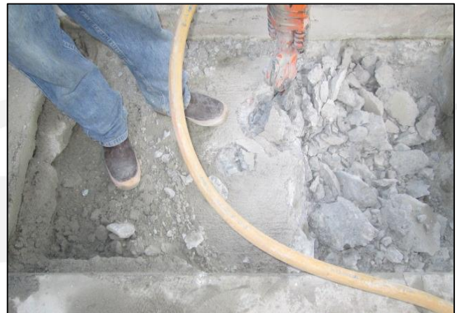
Pavement Under Soil Where AB Should Be (TYP)
