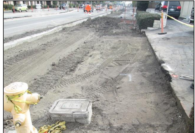
Rough Grade for DW at Grace and Carson
