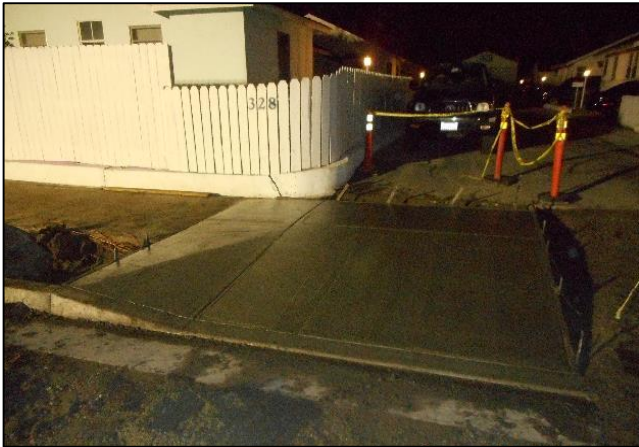
5500 PSI PCC Curing at 69+06.67 Prior to Broom Finish
