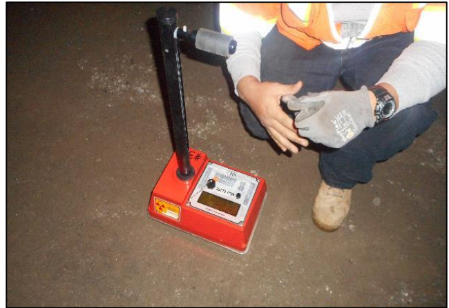
Checking Compaction at Driveway at Sta 78+75.89
