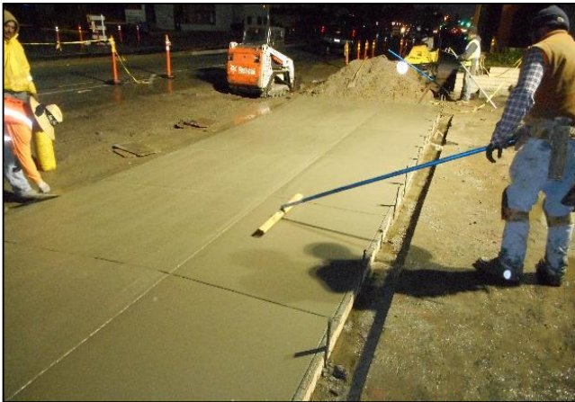
Broom Finishing 5500 PSI PCC at Driveway 67+26.28
