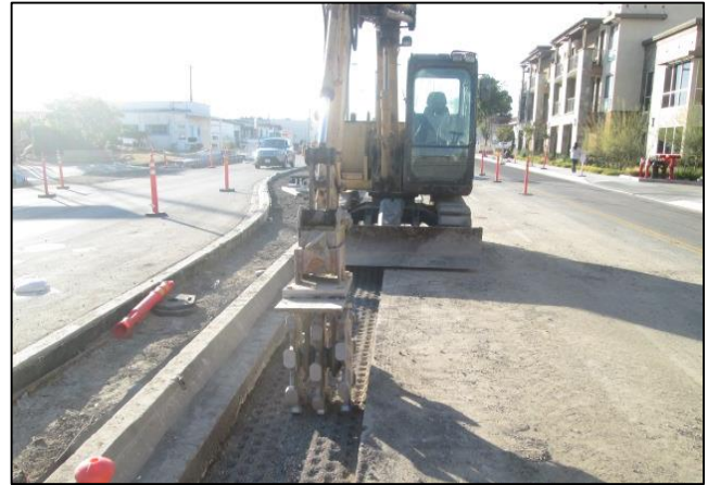
Compaction Wheel Used for Trench Backfill
