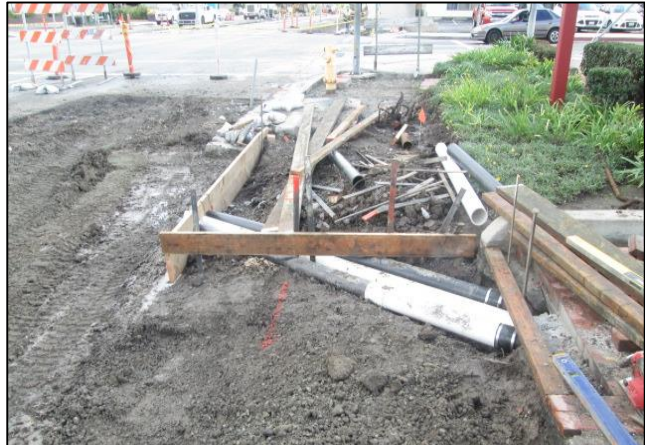
SCH 80 PVC Drains Under DW at 21713 Delores
