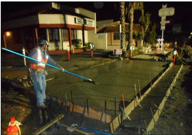
Finishing 5500 PSI PCC at Driveway Sta. 65+72.61
