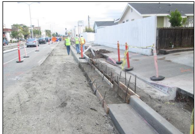
DW Curb Formed
