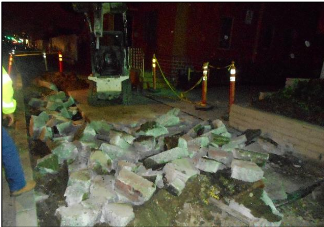
Concrete Broken for Removal
