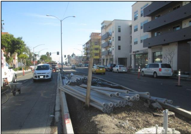
Conduit Stockpiled for Future Use
