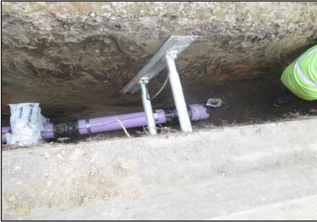
Water Line with 11.5 Degree Elbows Ready for Thrust Blocks
