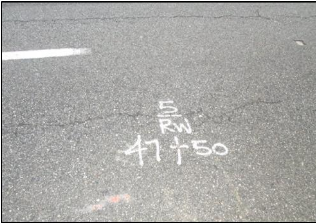
Station Marked with a Nail in the Street
