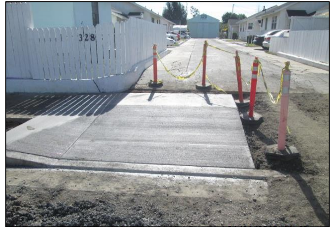
Driveway at 328 Carson
