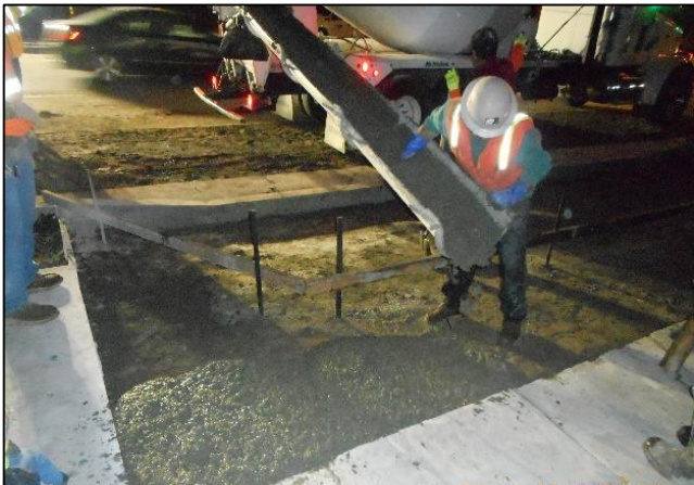
Placing 5500 PSI PCC at Driveway Sta. 78+75.89
