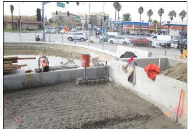
Drain at Fountain
