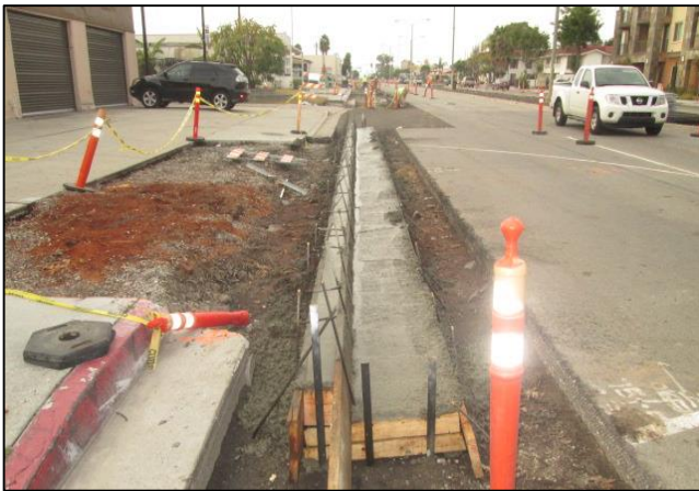
New Curb and Gutter Placement
