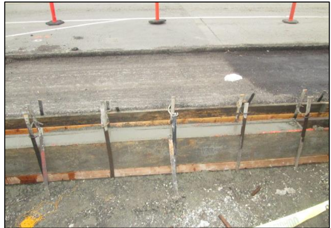
7" Curb and Gutter
