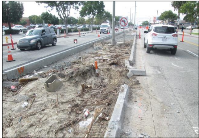
Median Curb Being Removed
